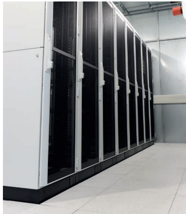
Amplifier room of the new hall
